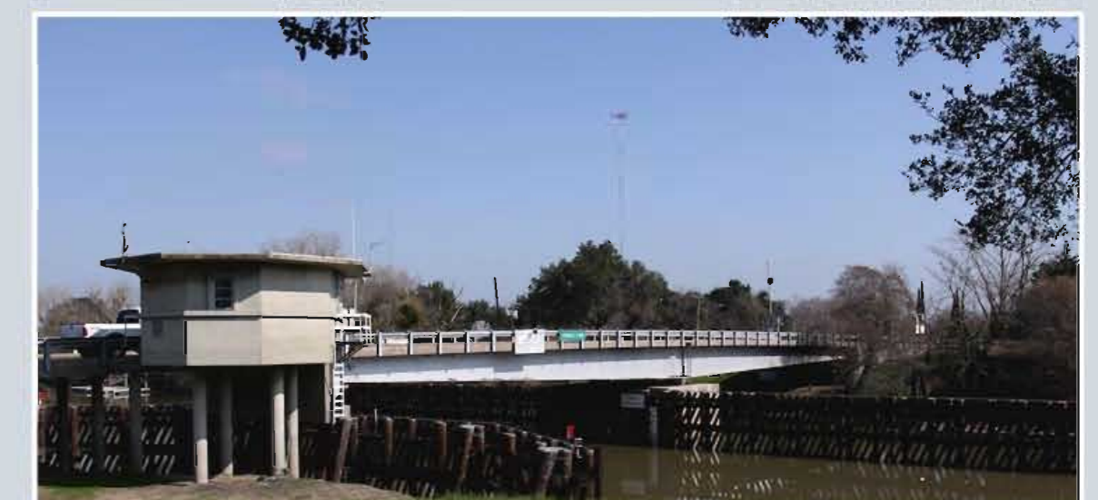
View looking approximately ENE of pier (www.bridgehunter.com)
