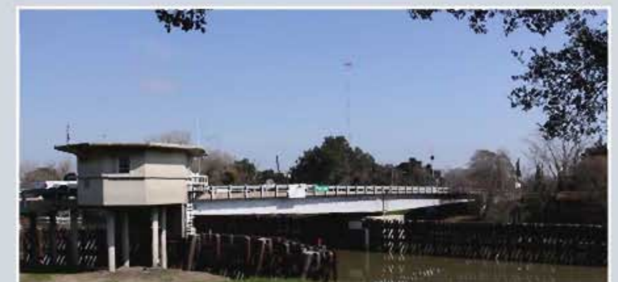
View looking approximately ENE of pier (www.bridgehunter.com)
