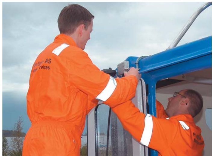
Mounting antennas on the wheelhouse
